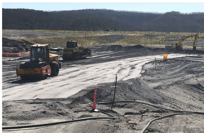
Above: Compaction of ash mixed with water at LNAR
